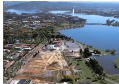
Clockwise from top left: Former Commonwealth Tank Farm Site, De-watering Discharge Treatment Pond, Aerial view of site
