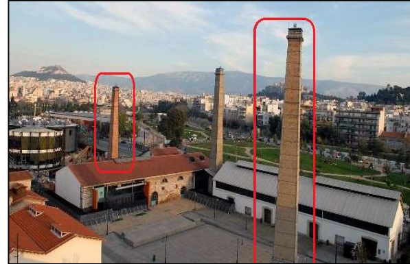
Figure 1. Chimneys A (left) and C (right) in Technopolis, Athens.
