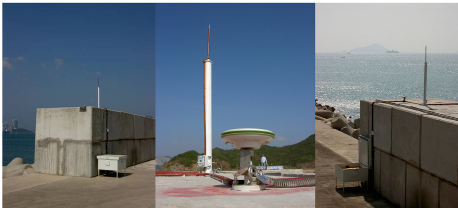
Figure 1: GPS monitoring antenna installed on a sea wall in Hong Kong.
