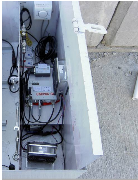
Figure 2: GPS receiver Leica GMX902 with power supply and communication interface.
