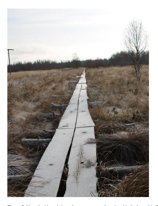
Figure 3. New duckboards have been constructed on the old plank road in Teuravuoma.
